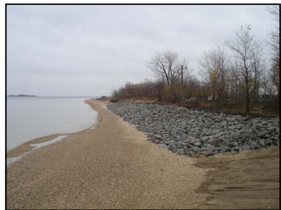
Shoreline protection project at Morris Point installed in 2008
